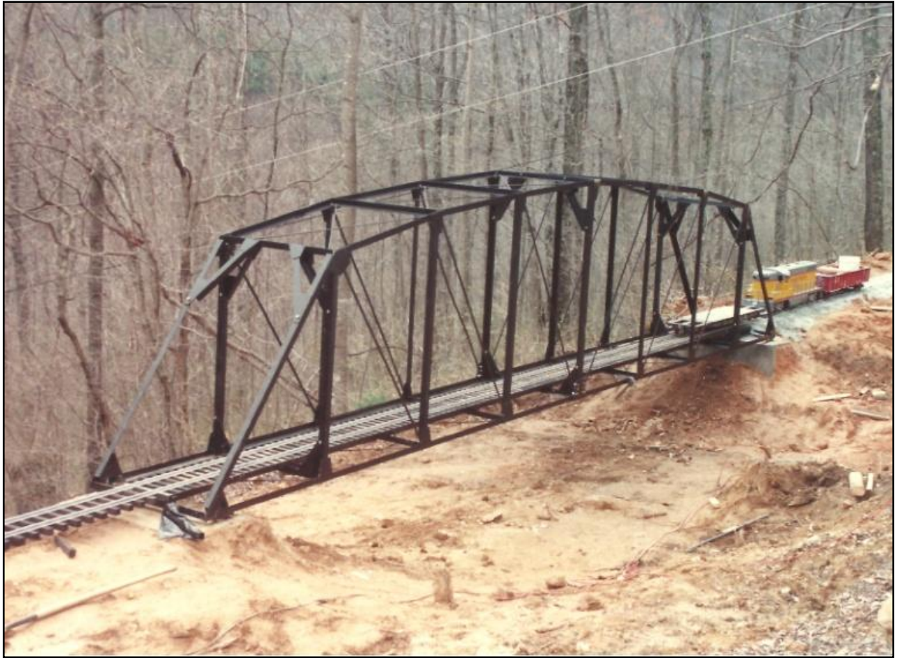
Tomm Tomlinson bridge, a 32' span
