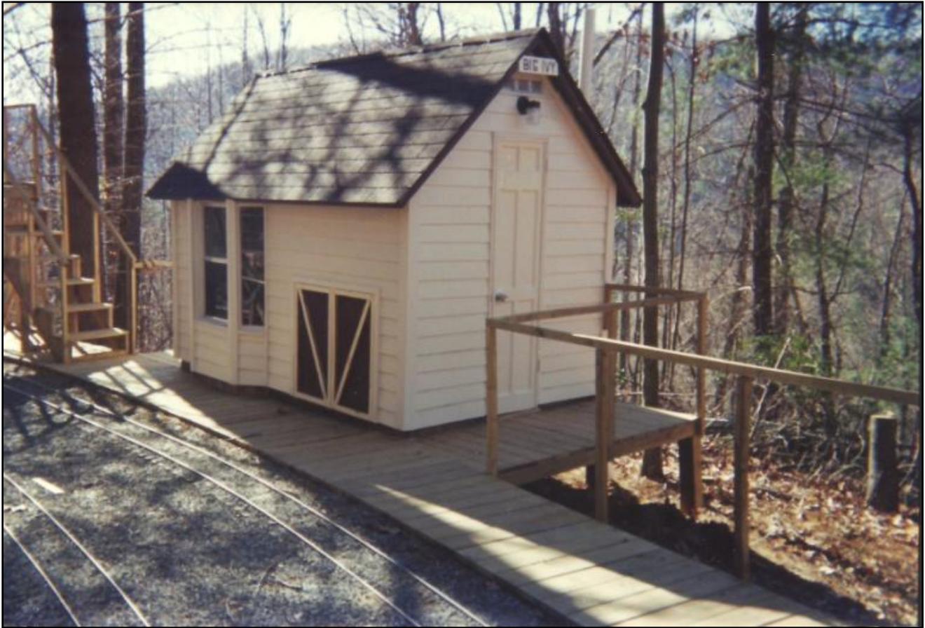
Big Ivy station overlooking the valley
